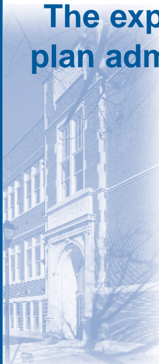
IMG World Headquarters Indianapolis, Indiana
